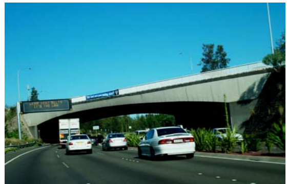
The VMS in this example detracts from the aesthetic qualities of the bridge. Increasing the separation between bridge and sign would produce a better composition of road elements.
