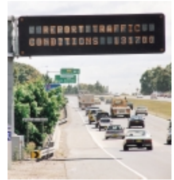
New M4 variable message signs give motorists up-to-the-minute information.
