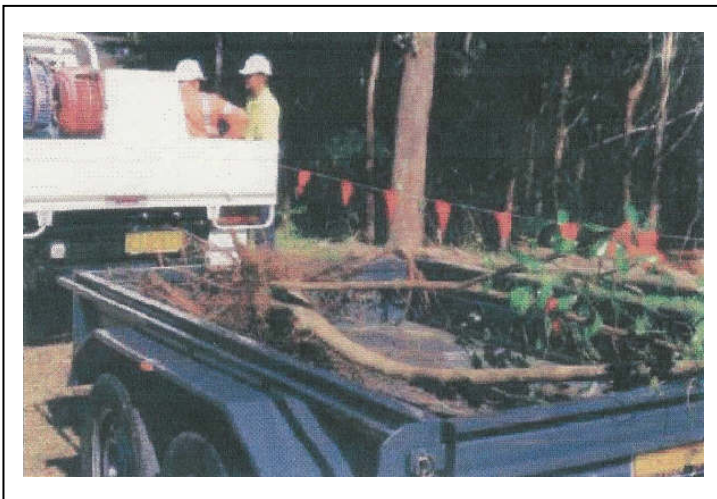
A Black Walnut (Endiandra Globosa) after being excavated on the Tugun bypass.
