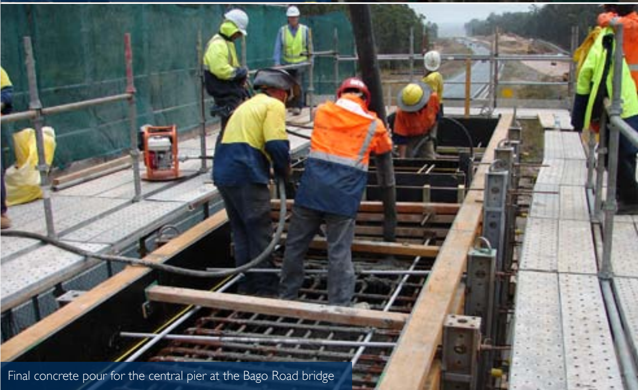
Placement of concrete at the abutment of Bago Road bridge
