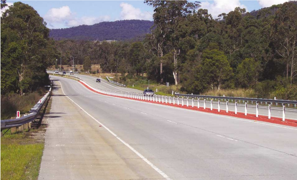
The photograph shows a wire rope installation on the Pacific Highway.
