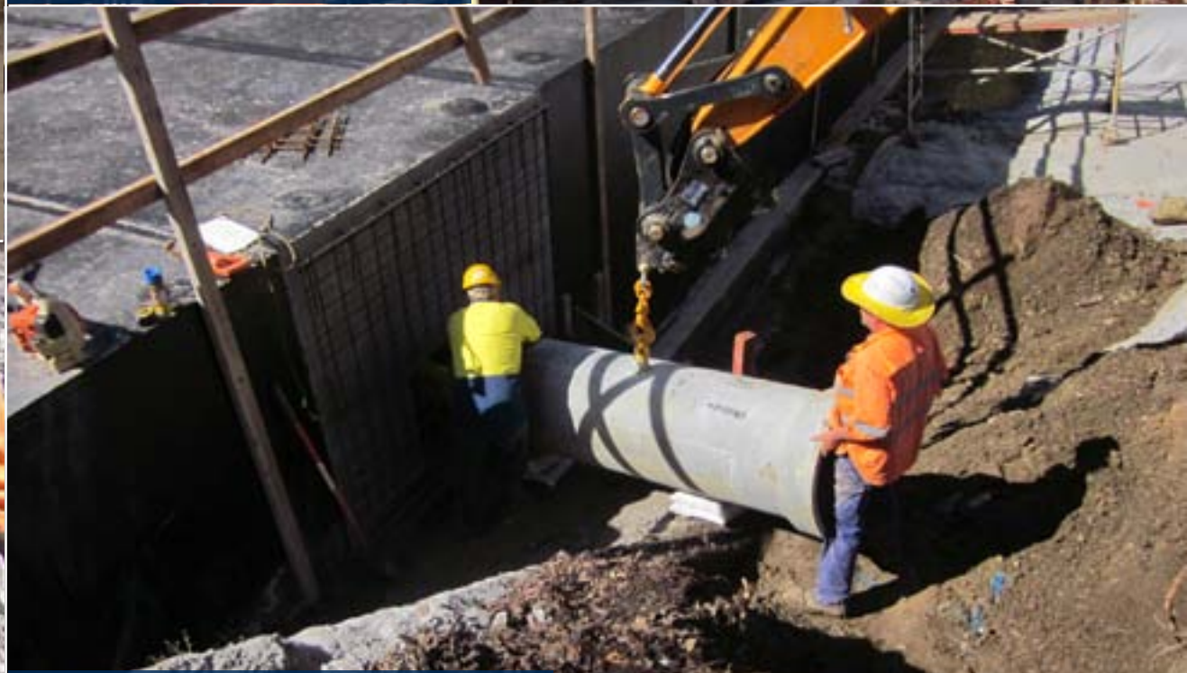
Pipe extension for the new northbound carriageway
