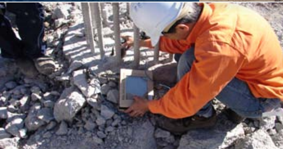
Pile integrity testing of abutment piles at Bago Road interchange
