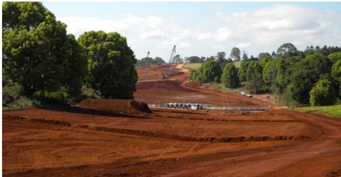
Bypass main alignment view east from Wollongbar.
